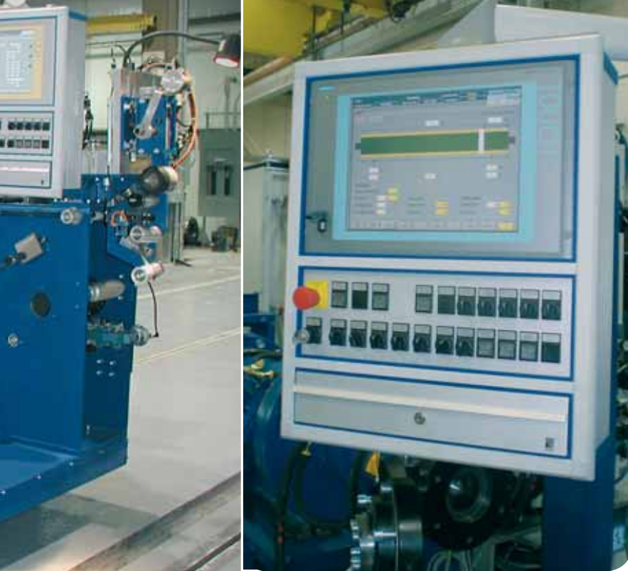
Central operator panel
